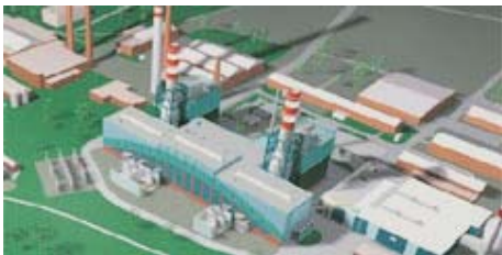
Kraftszer engineers were in charge of BOP of a combined cycle power plant
